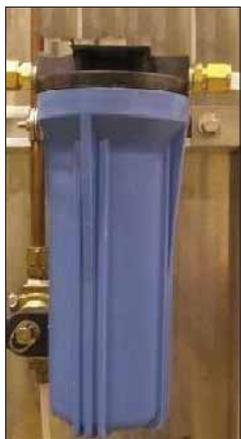
The filter 2 system, consisting of a molded carbon block filter (top) and housing (bottom), functioned on the principle of electrostatic attraction of negatively charged microorganisms to positively charged surfaces.
